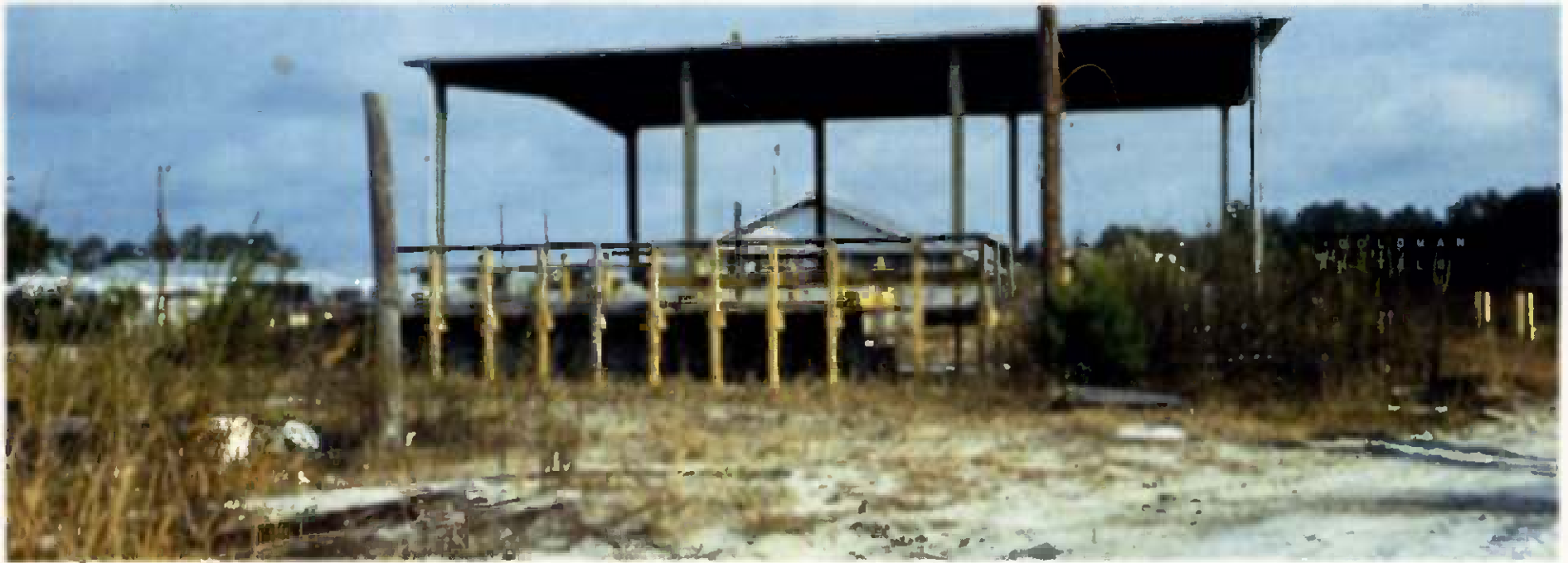
Photograph 2-3. Site 89, elevated wash rack (foreground), UST excavation area, and soil storage facility (background), looking north.
