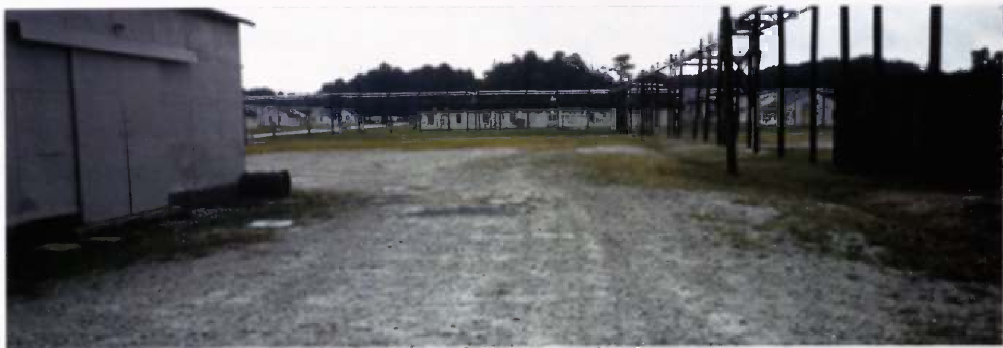
Photograph 3-2 Site 93, IIST excavation area and Building TC-942 (left), looking south
