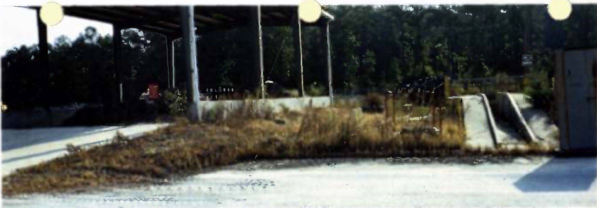
Photograph 2-1. Site 89, UST excavation area, soil storage building (left), and elevated wash rack (right), looking east.
