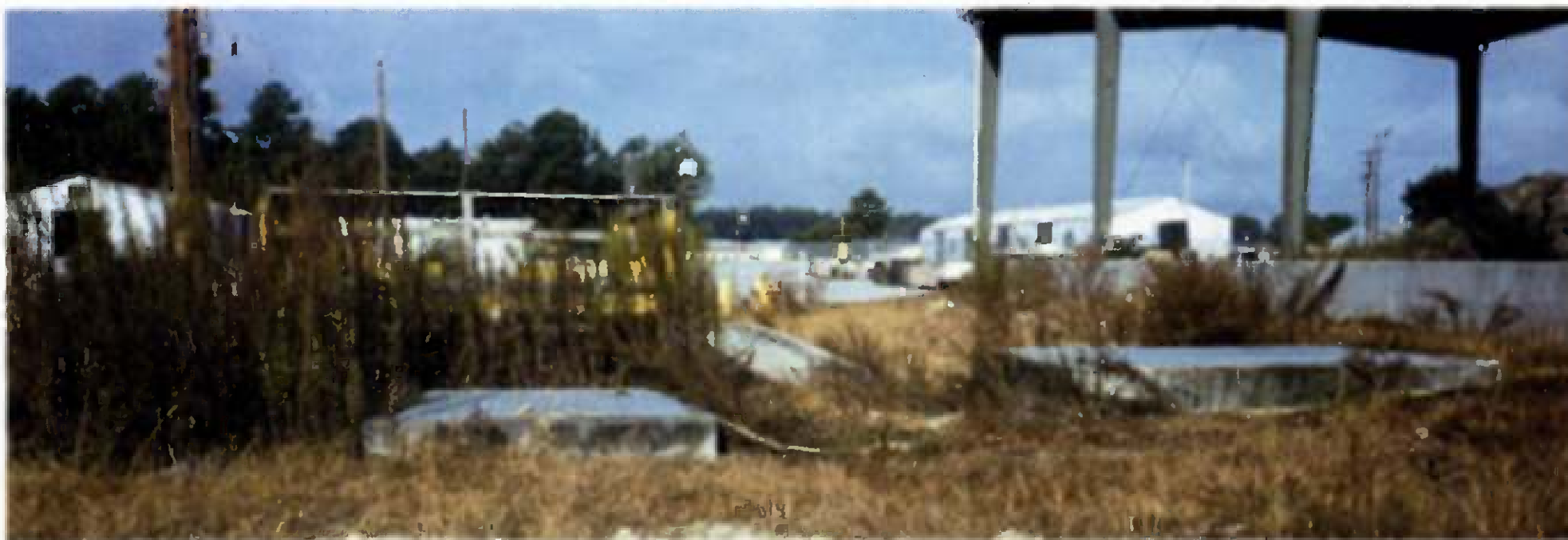
Photograph 2-2. Site 89, Oil/water separators (foreground) and UST excavation area, looking west.
