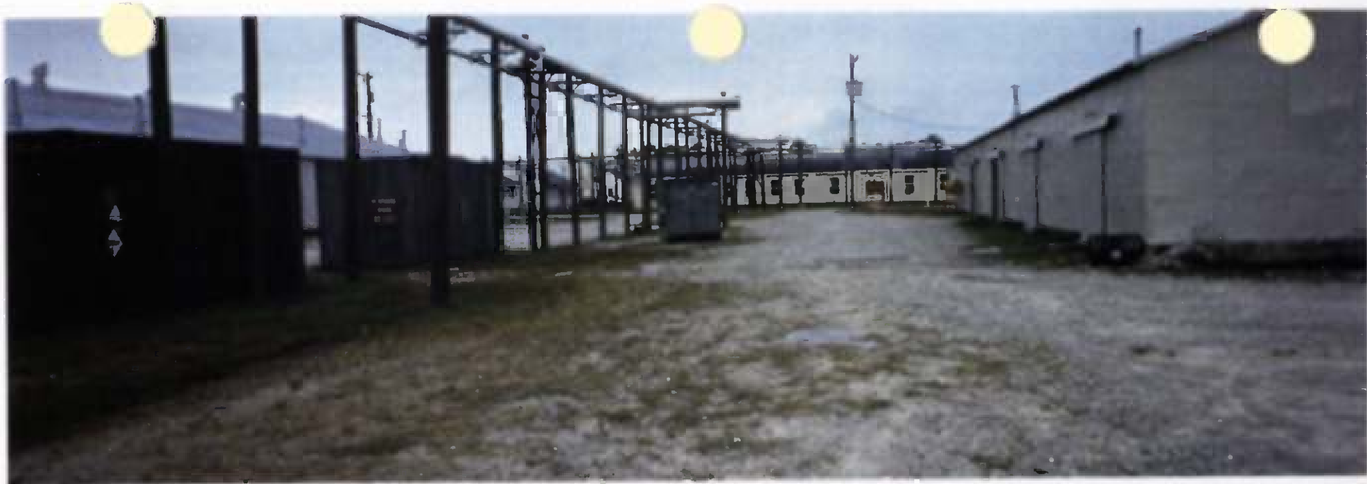
Photograph 3-1. Site 93, UST excavation area and Building TC-942 (right), looking north..
