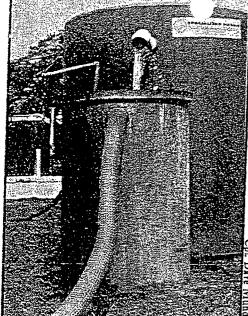
CLEANUP UNDERWAY— A pump and filter operate near the commissary in the Tarawa Terrace housing area, separating contaminants from groundwater. The housing area's water is supplied via a permanent line from the main water treatment plant on Holcomb Bouleyard.
