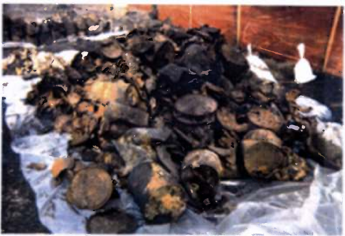
Project No. 15226 Contract No. N47408-92-D-3042 Delivery Order: 32 Location : north trenches Description: numerous containers (typical) excavated. containers in background - placed in roll-offs
