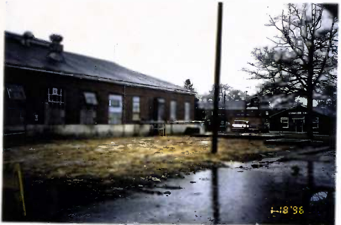
Project No. 17418 Date: 1/18/96 Contract No. N62470-93-D-3032 Delivery Order: 78 Location: Building 25 Description: Area after site restoration activities
