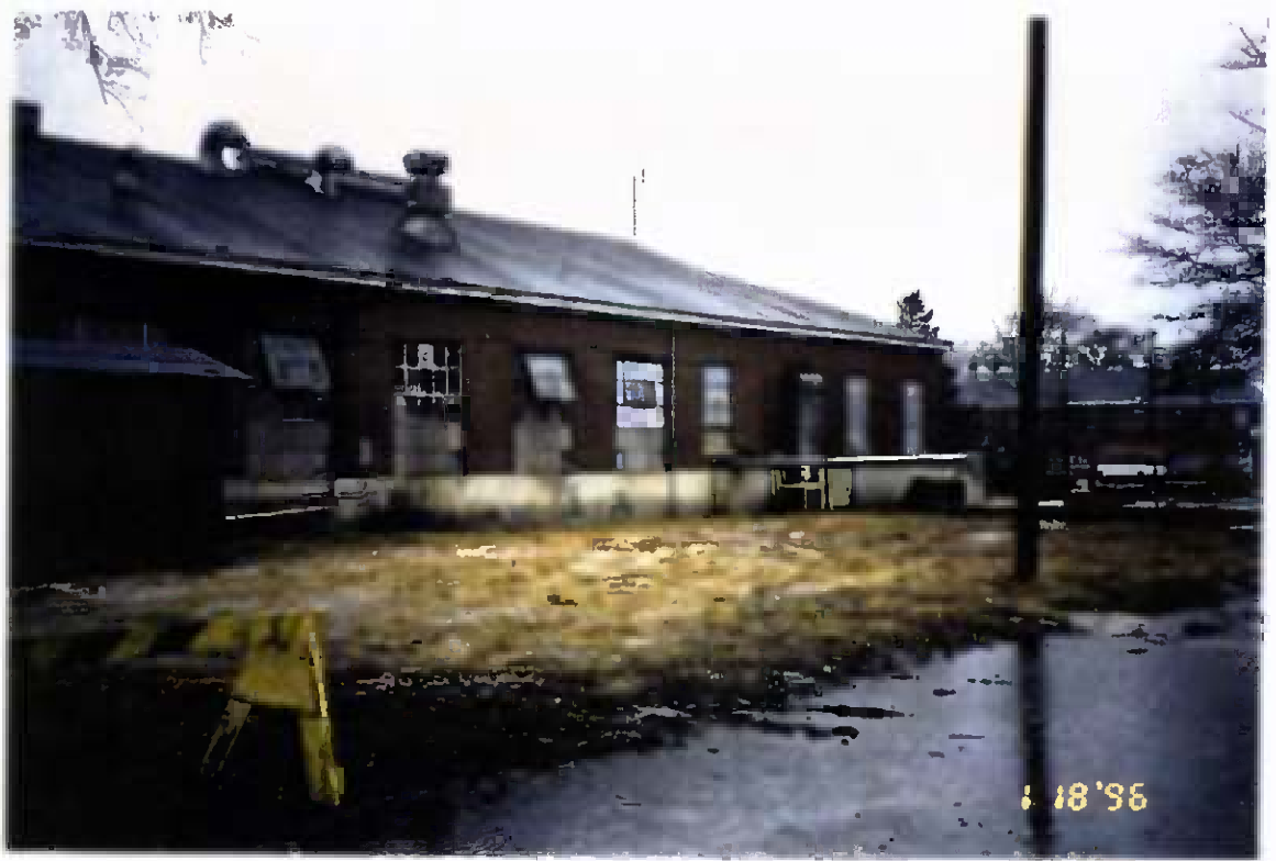
Project No. 17418 Date: 1/18/96 Contract No. N62470-93-D-3032 Delivery Order: 78 Location: Building 25 Description: Area after site restoration activities
