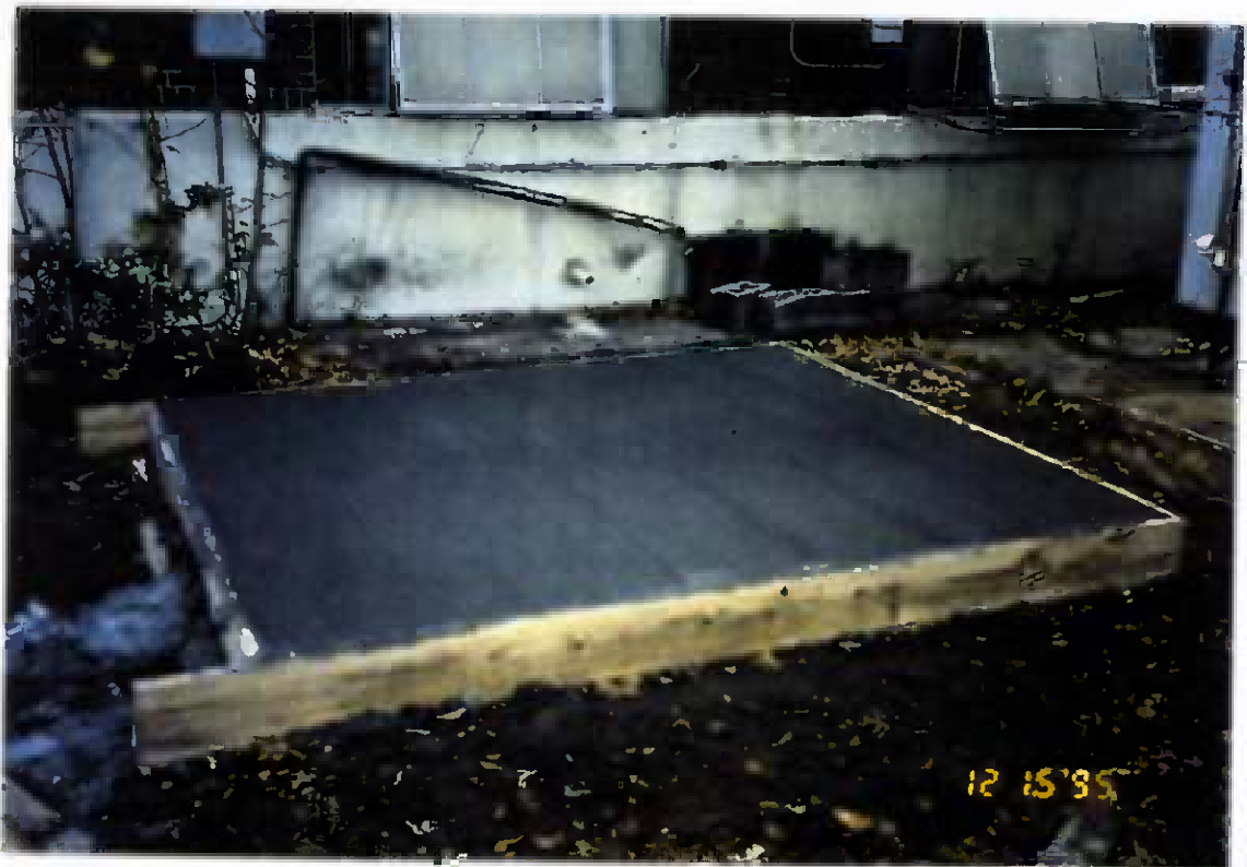
Project No. 17418 Date: 12/15/95 Contract No. N62470-93-D-3032 Delivery Order: 78 Location: Building 25 Description: Pad for air compressor
