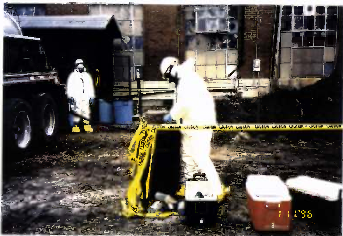
Project No. 17418 Date: 1/11/96 Contract No. N62470-93-D-3032 Delivery Order: 78 Location: Building 25 Description: Removal of tank contents into a tanker truck
