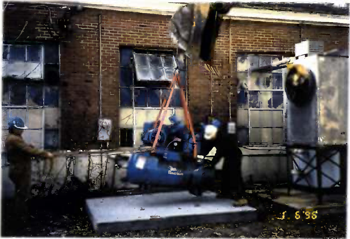
Project No. 17418 Date: 1/6/96 Contract No. N62470-93-D-3032 Delivery Order: 78 Location: Building 25 Description: Relocation of air compressor
