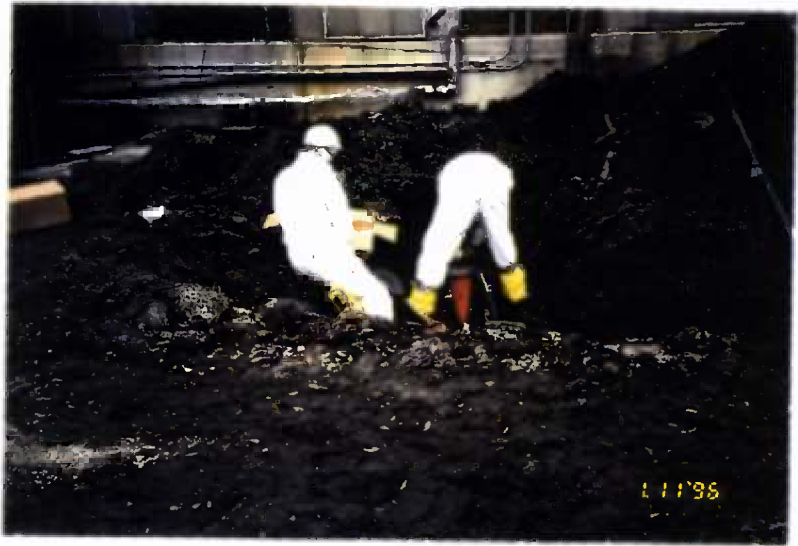
Project No. 17418 Date: 1/11/96 Contract No. N62470-93-D-3032 Delivery Order: 78 Location: Building 25 Description: Air monitoring from the tanks
