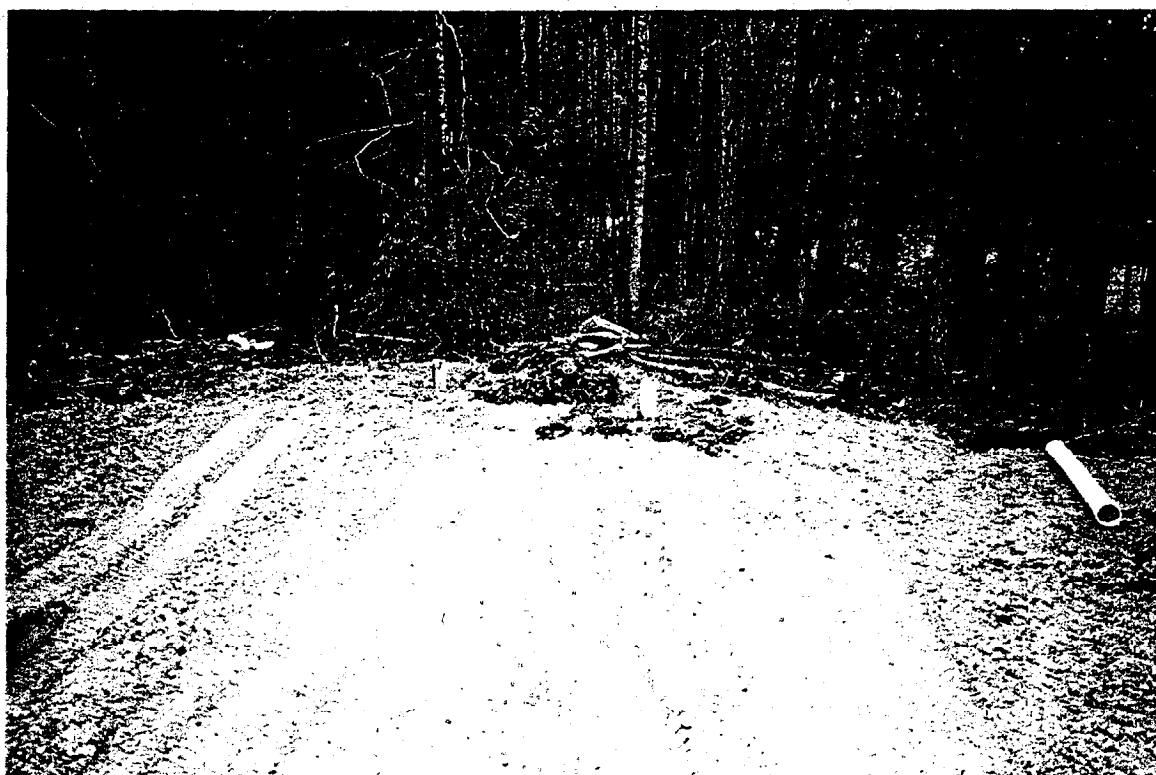
Project No. 17849 Date: 1/30/96 Contract No. N62470-93-D-3032 Delivery Order: 87 Location : Site 69 Description: temporary access road for well installation
