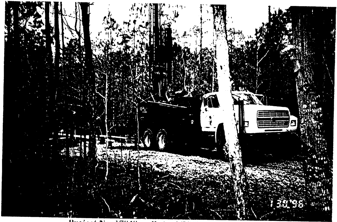
Project No. 17849 Date: 1/30/96 Contract No. N62470-93-D-3032 Delivery Order: 87 Location : Site 69 Description: temporary access road for well installation
