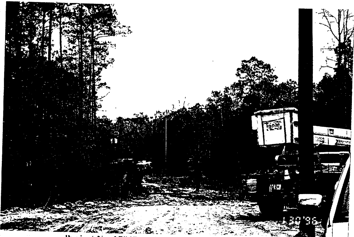
Project No. 17849 Date: 1/30/96 Contract No. N62470-93-D-3032 Delivery Order: 87 Location : Site 69 Description: power poles next to chemical dump area
