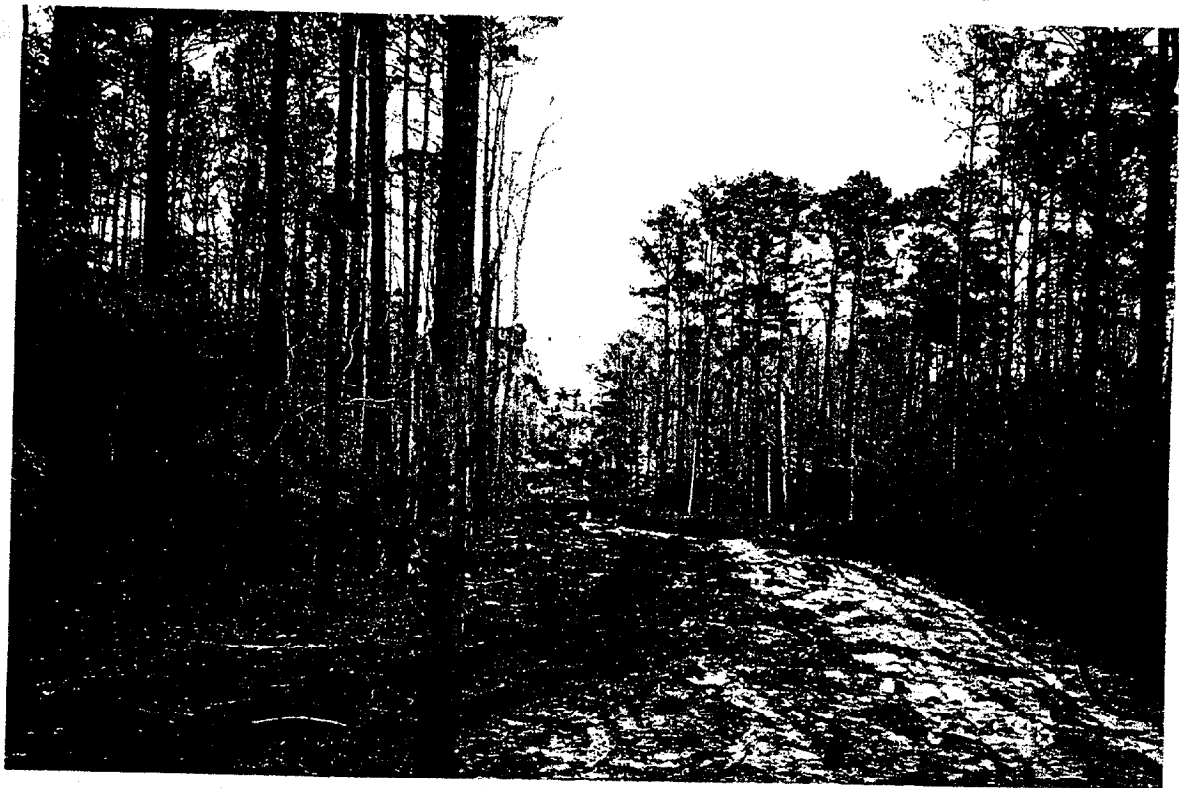
Project No. 17849 Date: 2/1/96 Contract No. N62470-93-D-3032 Delivery Order: 87 Location : Site 69 Description: cleared area for power poles
