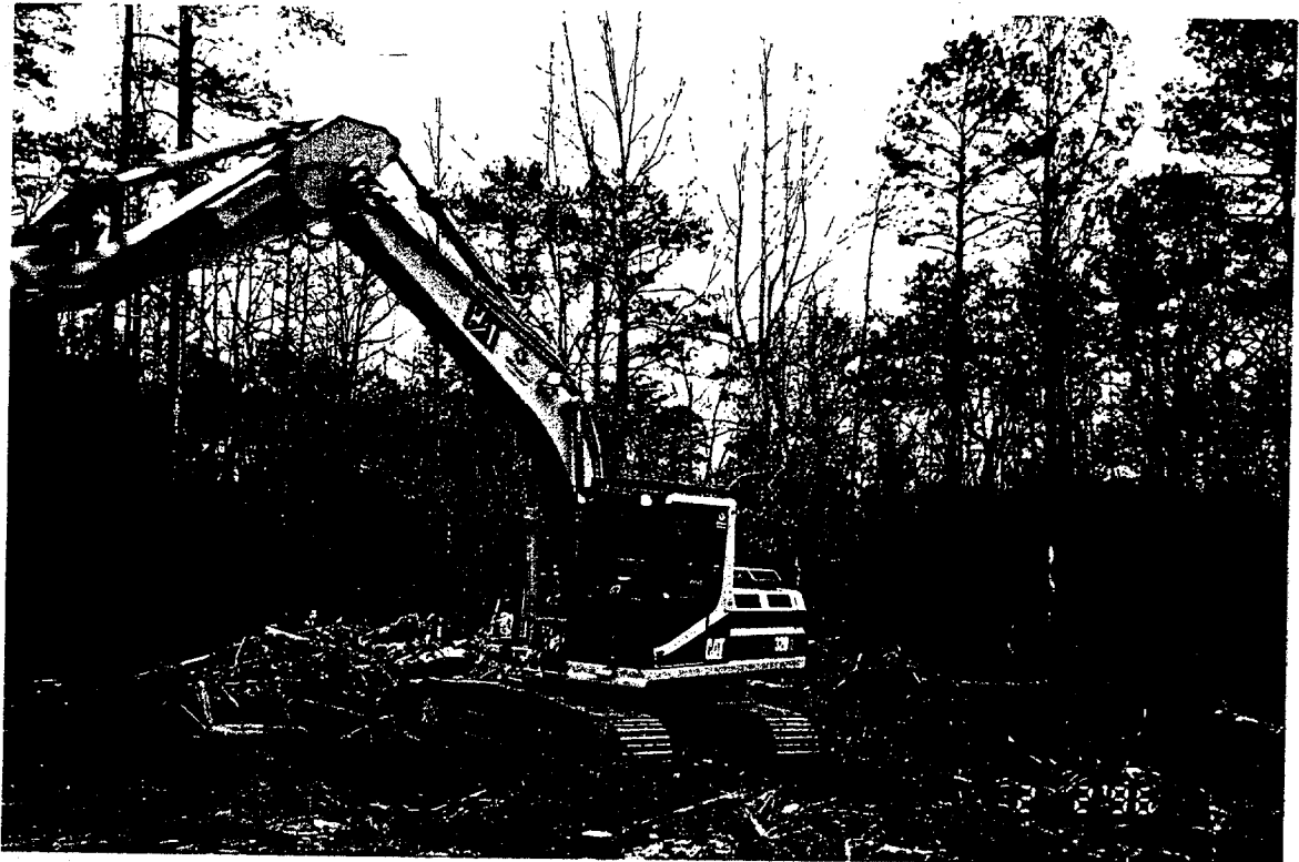
Project No. 17849 Date: 2/2/96 Contract No. N62470-93-D-3032 Delivery Order: 87 Location : Site 69 Description: clearing and grubbing
