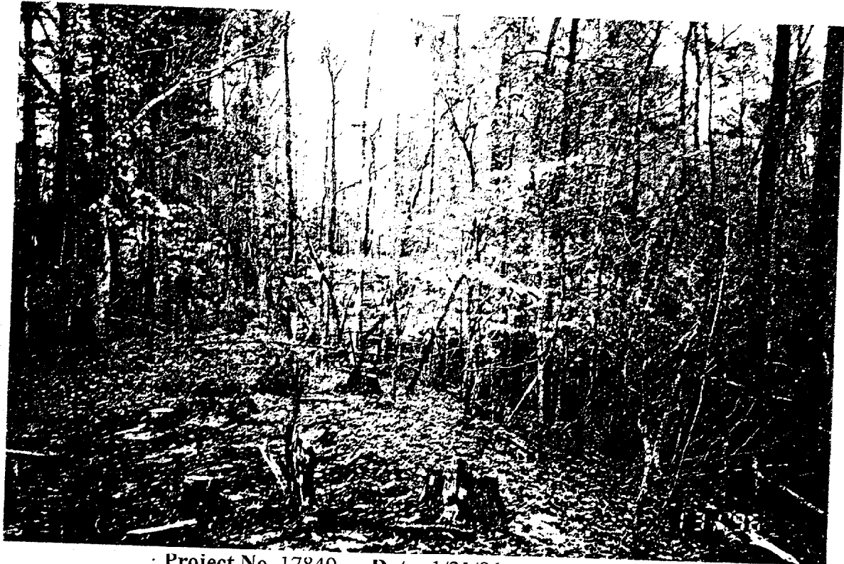
Project No. 17849 Date: 1/31/96 Contract No. N62470-93-D-3032 Delivery Order: 87 Location : Site 69 Description: clearing and grubbing
