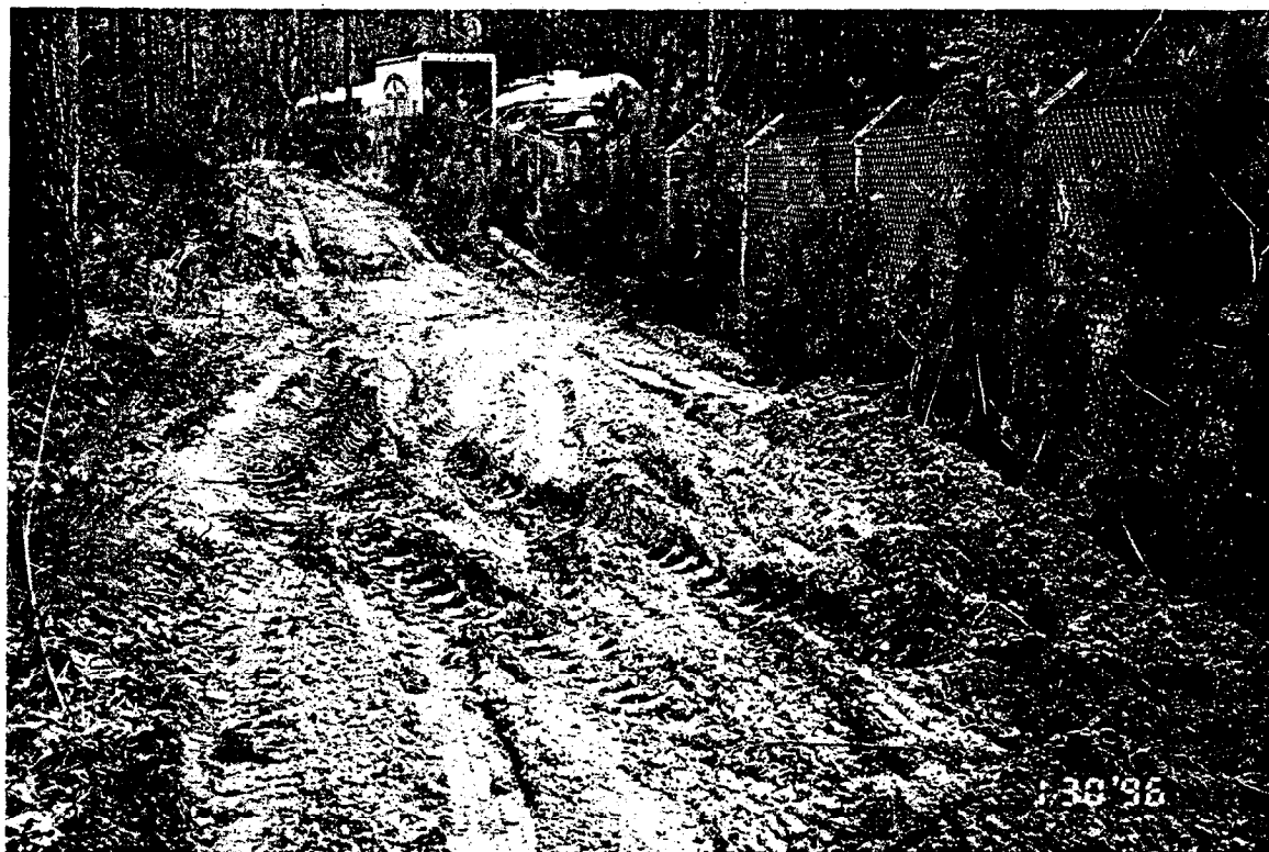
Project No. 17849 Date: 1/30/96 Contract No. N62470-93-D-3032 Delivery Order: 87 Location : Site 69 Description: temporary access road for well installation
