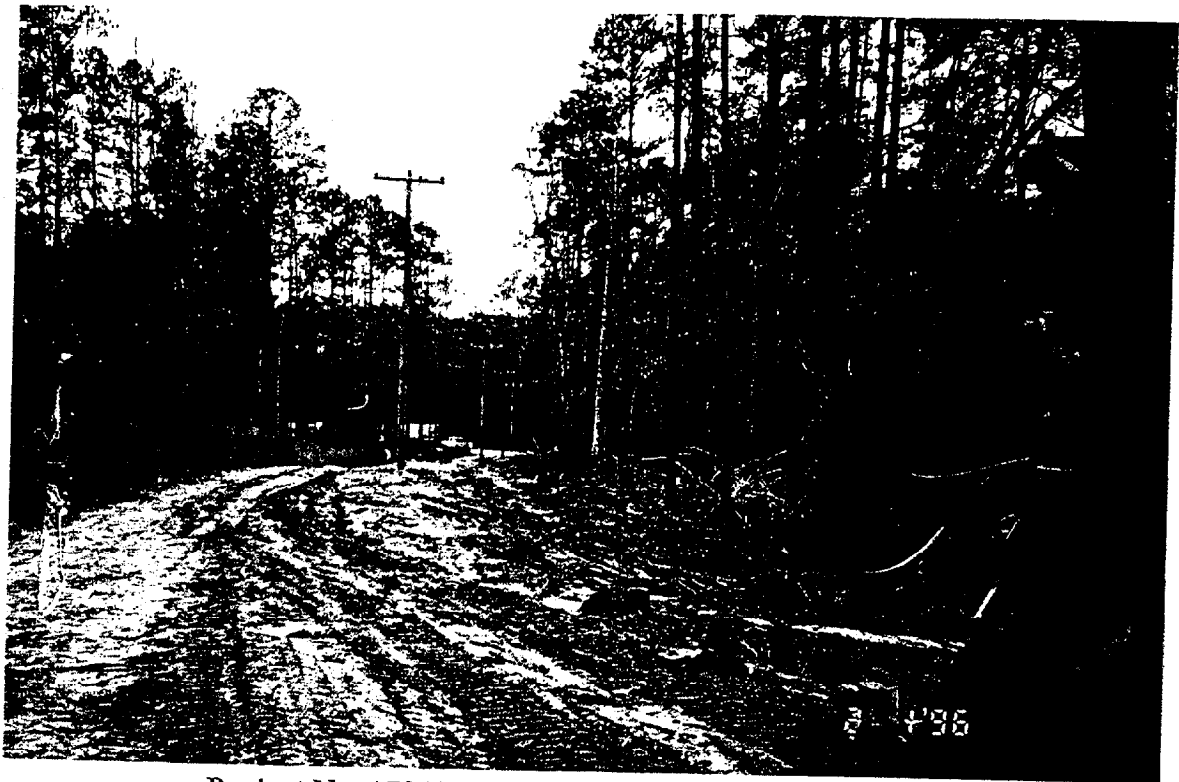
Project No. 17849 Date: 2/1/96 Contract No. N62470-93-D-3032 Delivery Order: 87 Location : Site 69 Description: power poles installed on chemical dump side
