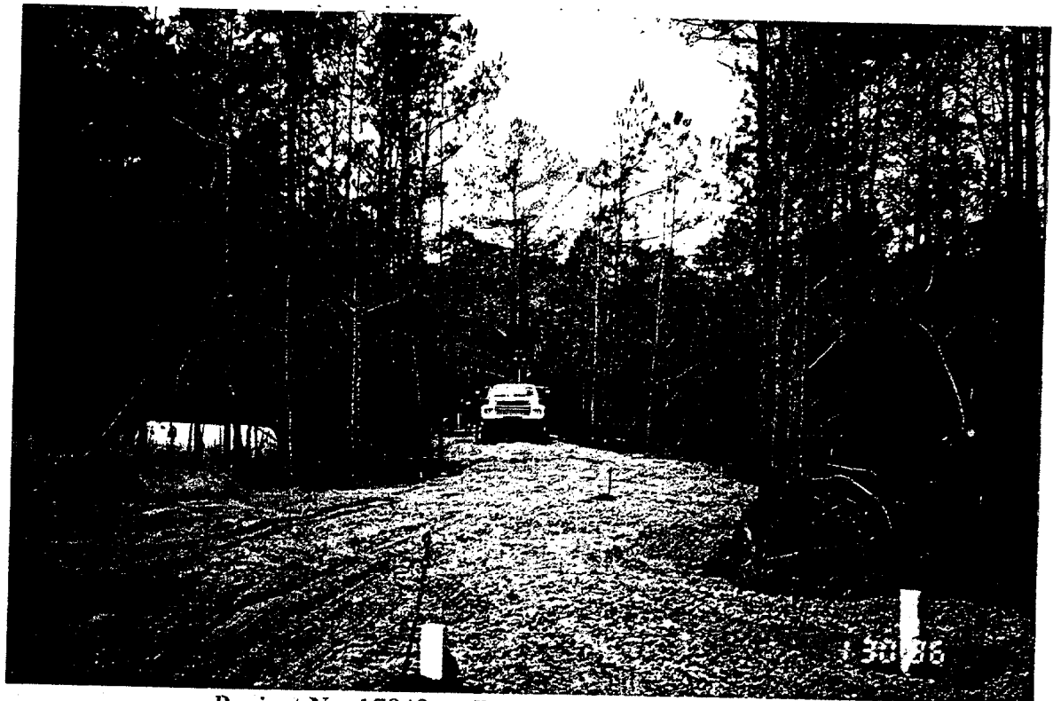
Project No. 17849 Date: 1/30/96 Contract No. N62470-93-D-3032 Delivery Order: 87 Location : Site 69 Description: temporary access road for well installation
