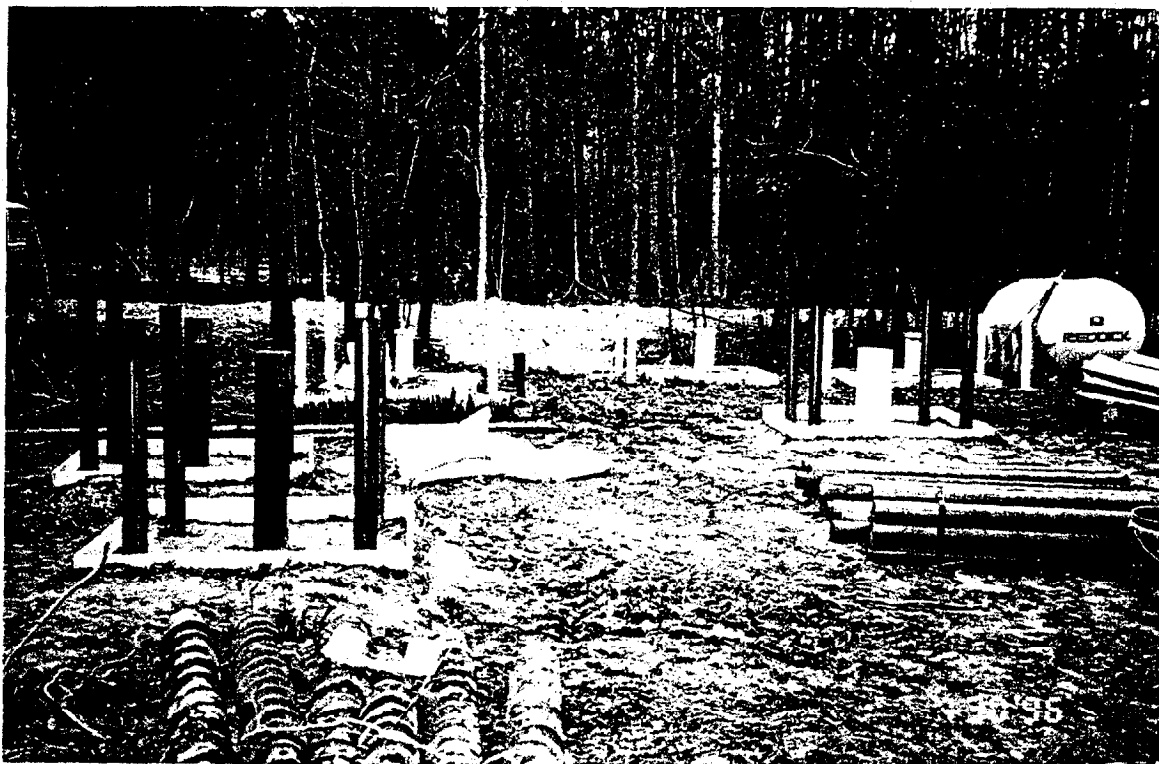
Project No. 17849 Date: 1/30/96 Contract No. N62470-93-D-3032 Delivery Order: 87 Location : Site 69 Description: temporary access road for well installation
