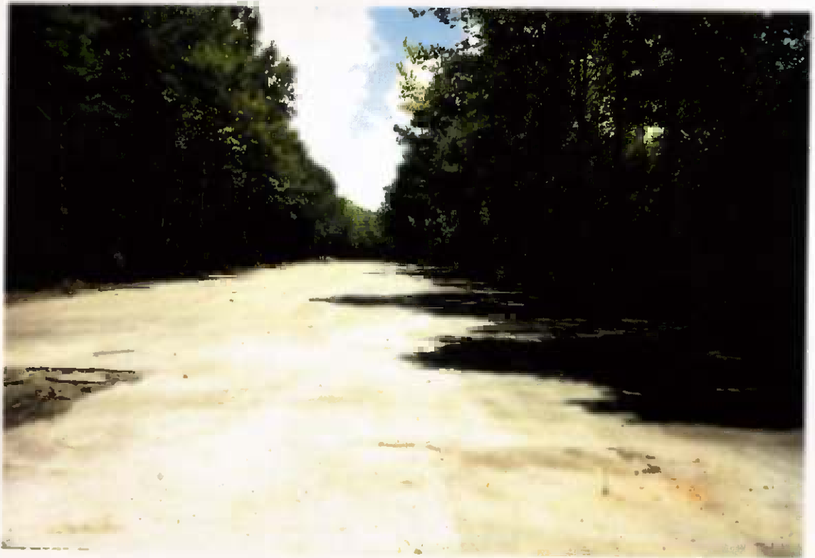
Project No. 16487 Date: 7/28/95 Contract No. N62470-93-D-3032 Delivery Order: 44 Location: Contaminated Stockpile Area Description: Area after cleaning
