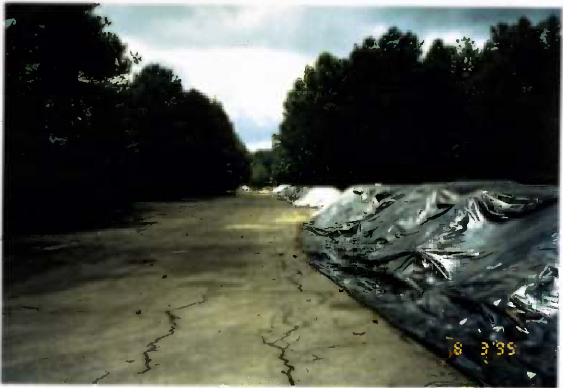
Project No. 16487 Date: 8/3/95 Contract No. N62470-93-D-3032 Delivery Order: 44 Location: Contaminated stockpile area Description: Covered stockpiled soils
