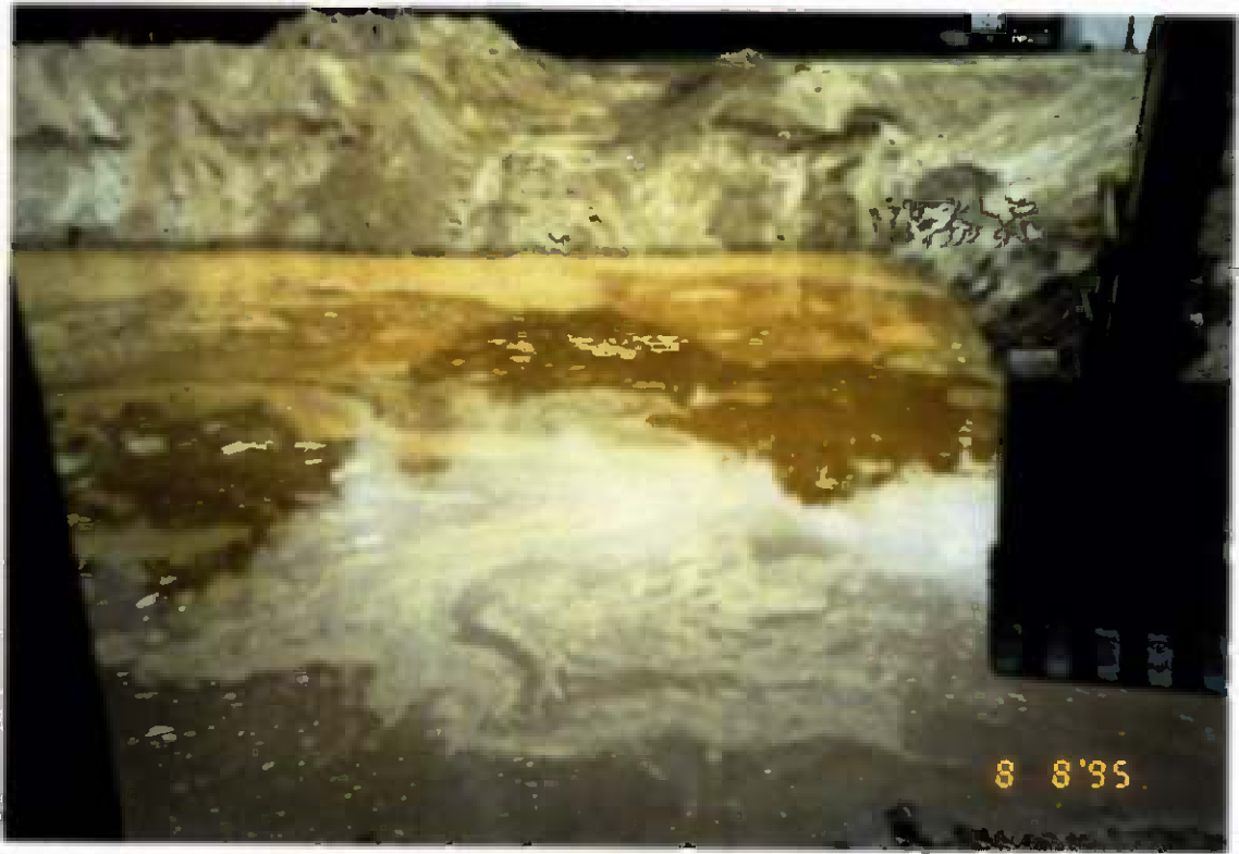
Project No. 16487 Date: 8/8/95 Contract No. N62470-93-D-3032 Delivery Order: 44 Location: Area C Description: Groundwater ponding
