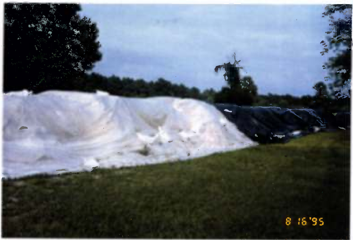
Project No. 16487 Date: 8/16/95 Contract No. N62470-93-D-3032 Delivery Order: 44 Location: Contaminated soil staging area Description: Secondary staging area totally full
