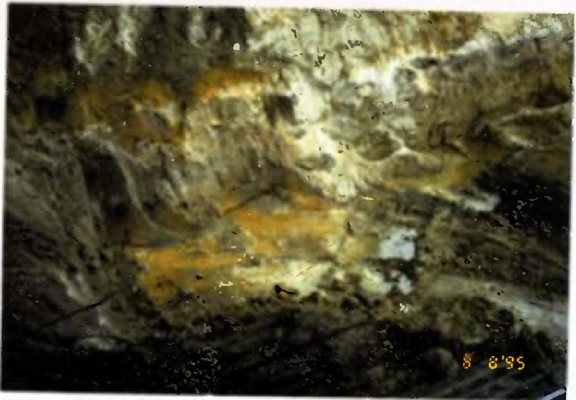
Project No. 16487 Date: 8/8/95 Contract No. N62470-93-D-3032 Delivery Order: 44 Location: Area C Description: Showing visible contamination
