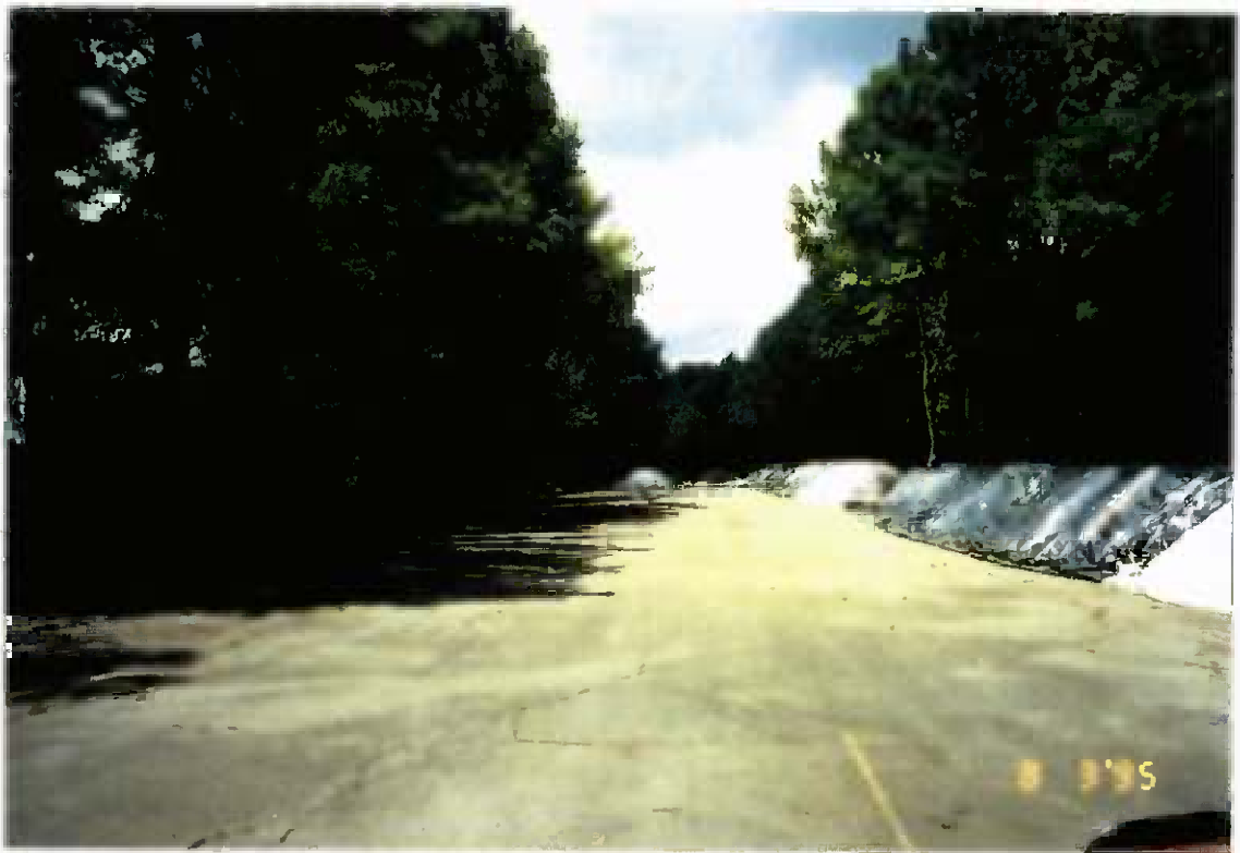
Project No. 16487 Date: 8/3/95 Contract No. N62470-93-D-3032 Delivery Order: 44 Location: Contaminated soil staging area Description: Contaminated soil staging area
