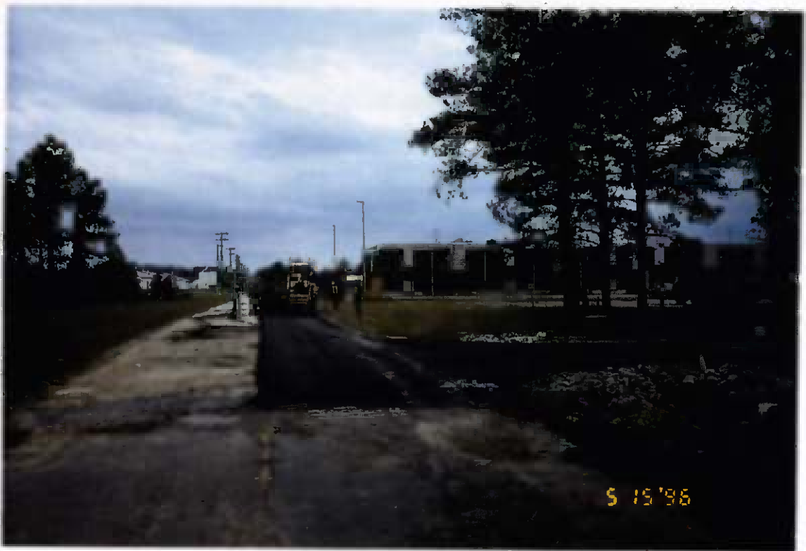
Project No. 16487 Date: 5/15/96 Contract No. N62470-93-D-3032 Delivery Order: 44 Location: 'F' Street - Camp Geiger Description: Placing asphalt paving
