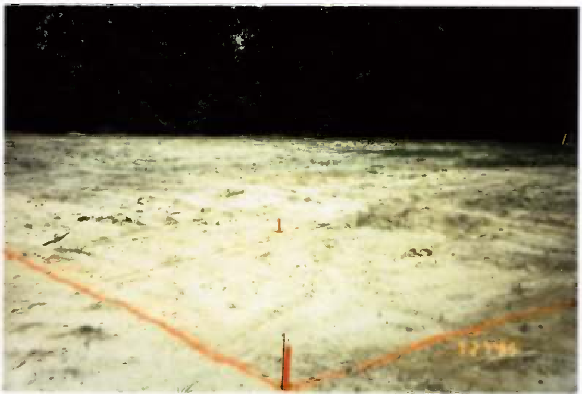
Project No. 16487 Date: 7/27/95 Contract No. N62470-93-D-3032 Delivery Order: 44 Location: Area C Description: Pre-excavation grid
