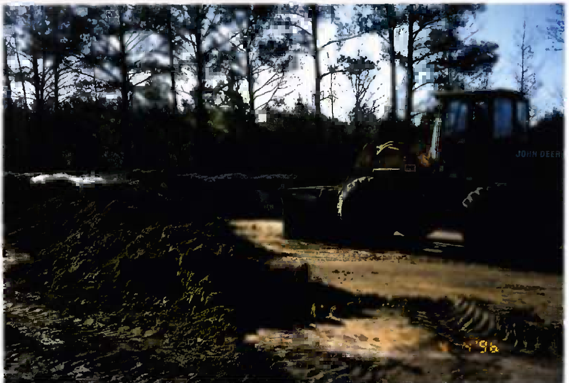
Project No. 16487 Date: 4/4/96 Contract No. N62470-93-D-3032 Delivery Order: 44 Location: Contaminated soil area Description: Loading out TPH contaminated soil
